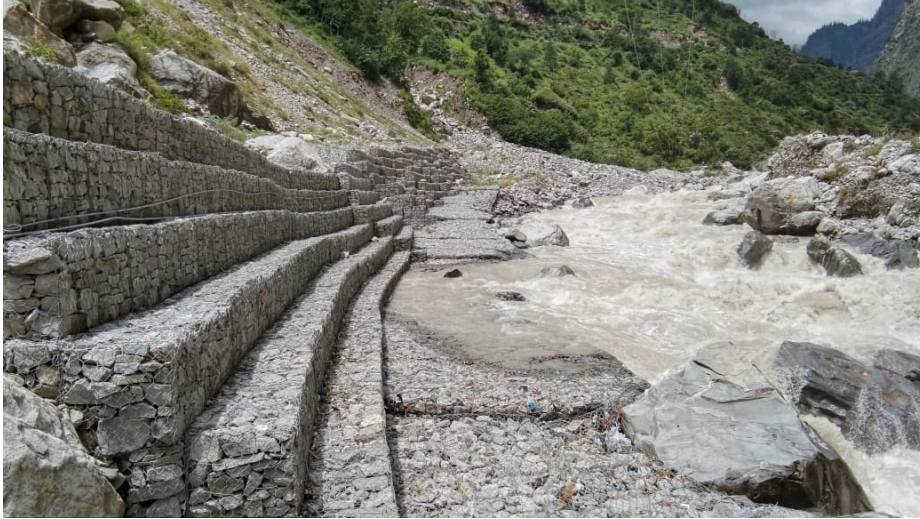
Fig. 21. Photograph showing the bank protection works adopted at site
