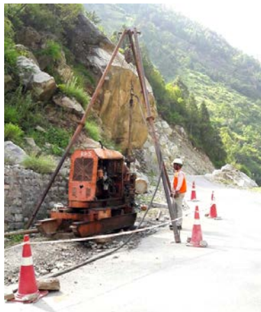
Fig. 4. Borehole drilling in progress
